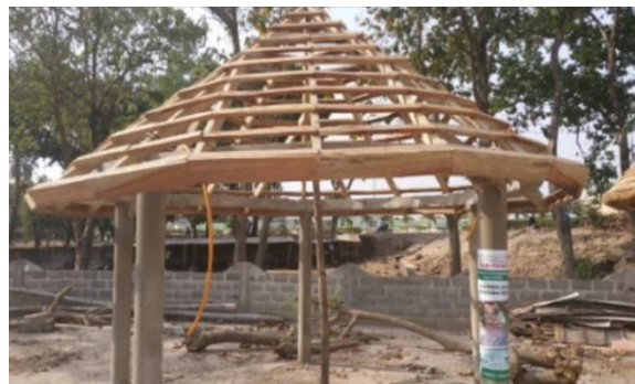
Fig. 3: Wood frames for straw roof
