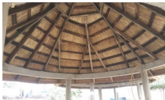
Fig. 2: Interior view of straw roof
