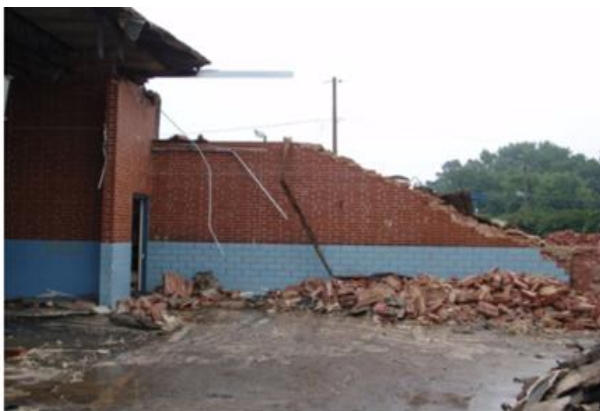
(b) After demolition
