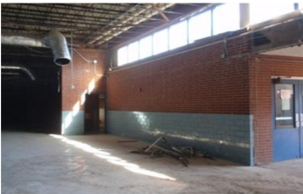
(a) Before demolition
